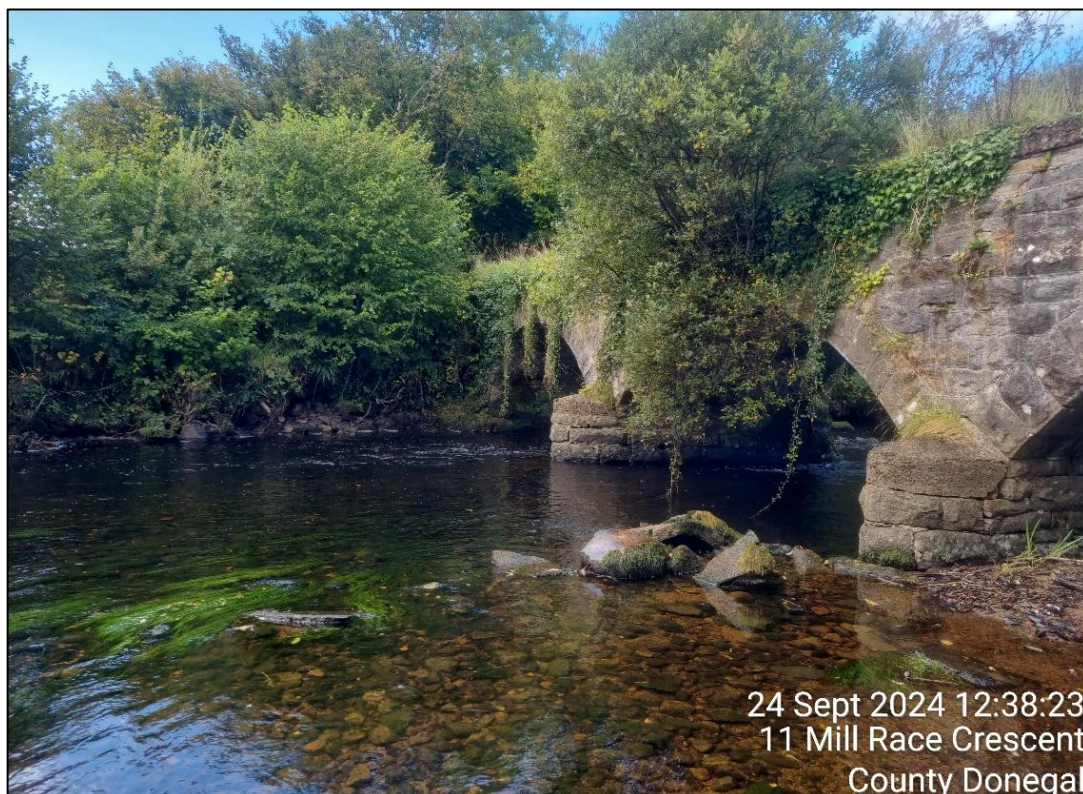
Figure 7-2 - Depositing/lowland rivers (FW2) habitat at existing River Eske crossing in Donegal Town (Ch. 750)
